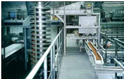
Figure 4: Vibrating spiral conveyors and trough conveyors in a food processing factory
